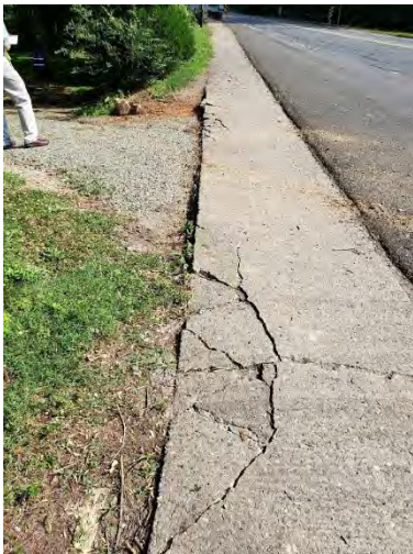
Cracked sidewalk, Route 1 (a)
