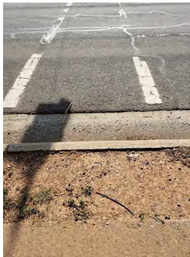
Crosswalk no curb cuts, sparse paint, Route 1(e)
