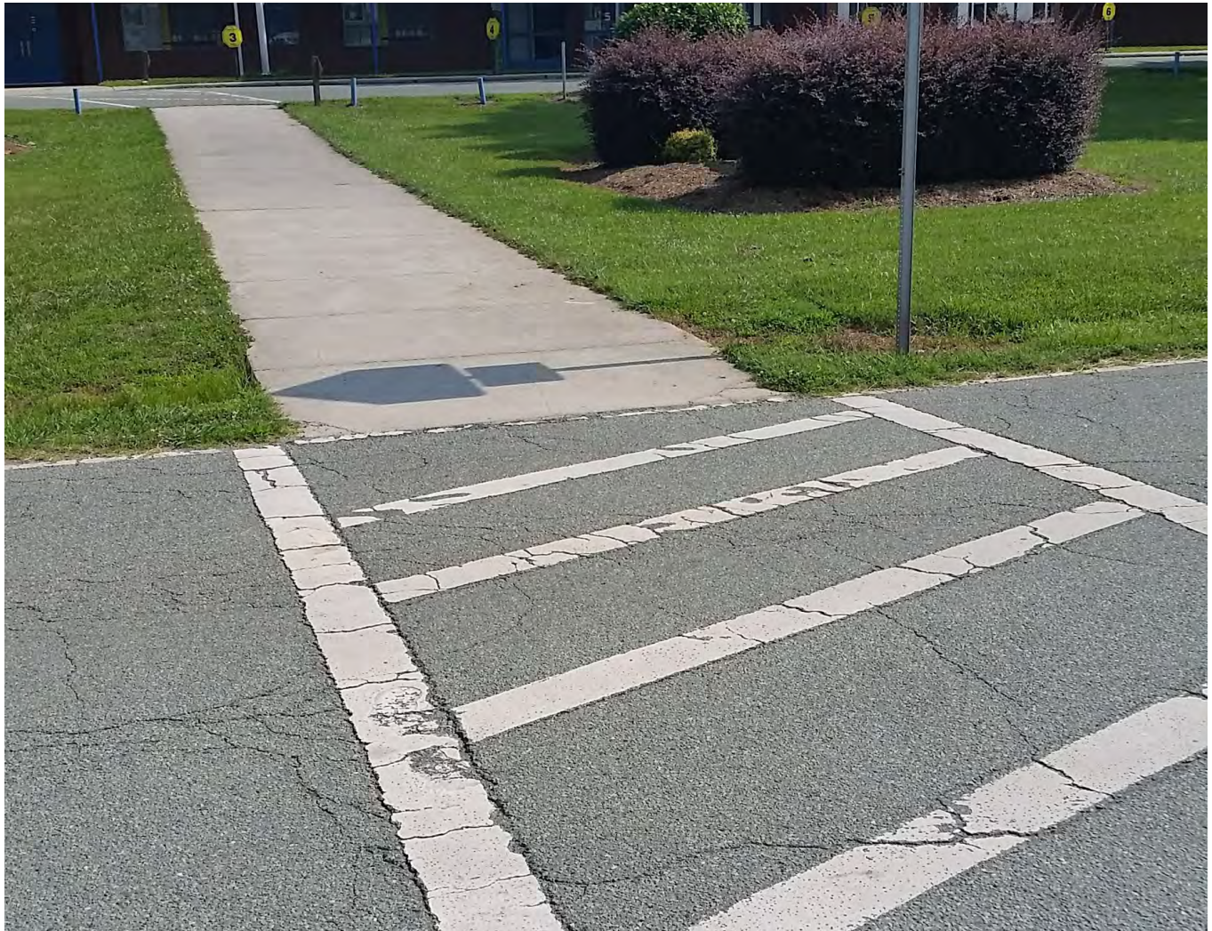
Existing crosswalk leading from the parking lot driveway to the sidewalk entrance to Pittsboro Elementary School.
